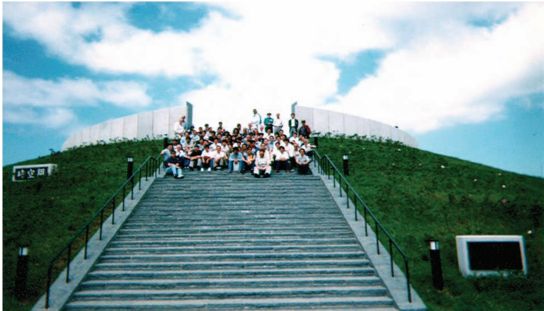
Figure A-5 Berm constructed for tsunami refuge in Aonae, Japan.
