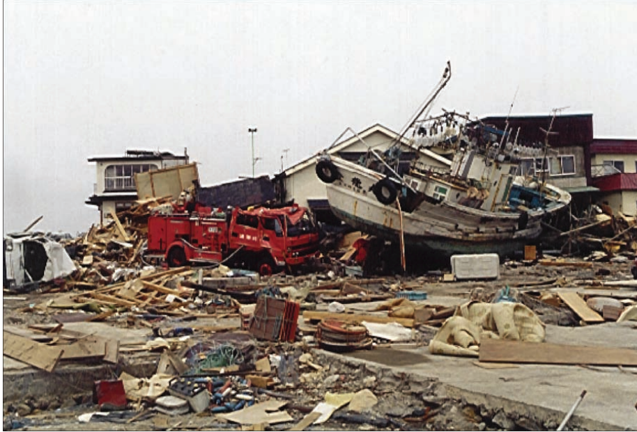
Figure 2-12 Damage caused by impact from water-borne debris (fishing boat) in Aonae, Japan (1993 Okushiri Tsunami) (Photo courtesy J. Preuss).
