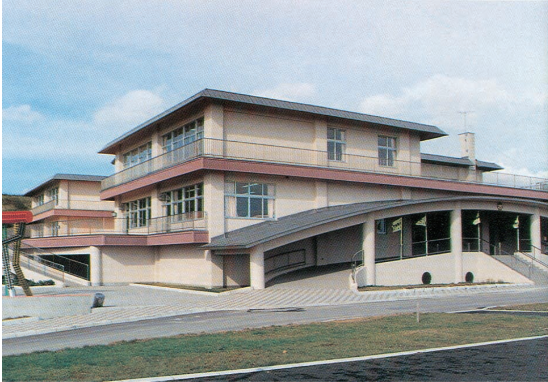
Figure A-6 Aonae Elementary School. Upper floors are intended for use as tsunami refuge space.
