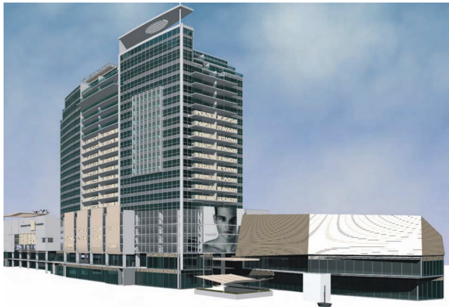
Figure 4-4 Hotel and convention complex. Meeting rooms, ballrooms, and exhibit spaces located above the tsunami inundation elevation can be used to provide areas of refuge.
